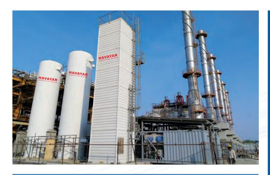
Havayar Cryogenic Air Separation Technology are designed for production of Liquid and/ or Gases Oxygen, Nitrogen & Argon from Atmospheric Air based on the low-temperature Rectification process. Our Cryogenic Air Separation Plant produce tons of  $O_2$ ,  $N_2$  & AR efficiently and safely 24 hr/day, 7 days/week, 365 days/year. We offer our products under license of ASME, DIN, EN, API, European Standard & IEC.
